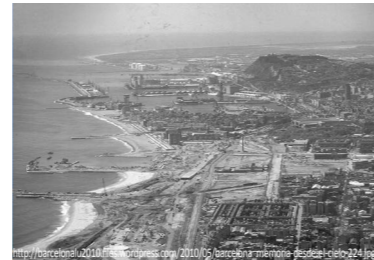
Waterfront under construction. It was mainly industrial use and not accessible to the public..
